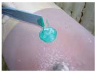
10. Dispense the desired amount of mixed material onto the clean area and spread it immediately over the patch/damage area, using a spatula or suitable tool.
