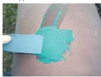
Apply the material to a uniform thickness immediately, while the material is wet.
