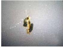
2. Clean the damaged/patch area by removing the loose coating, dust and other contaminants.
