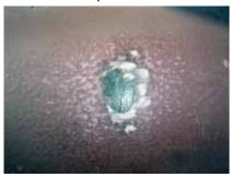
4. Clean the steel surface, so that rust is completely removed. Additionally the surface must be clean of grease, oil, salts and other contaminants. If necessary, wipe/clean the area with Acetone, MEK or other suitable solvent which does not leave a residue. Remove all moisture from the area to be repaired.
