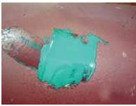
12. Allow the repaired/coated area to cure. The repaired/coated area should be protected from any accidental damage until the epoxy has completely cured. Powercrete R-65/F1 is a fast cure epoxy. Check cure time chart for cure values
