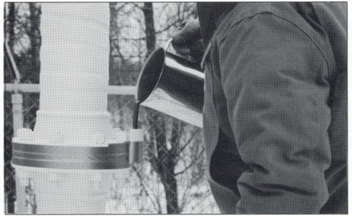
Innercoat being used in a horizontal flange fill.
