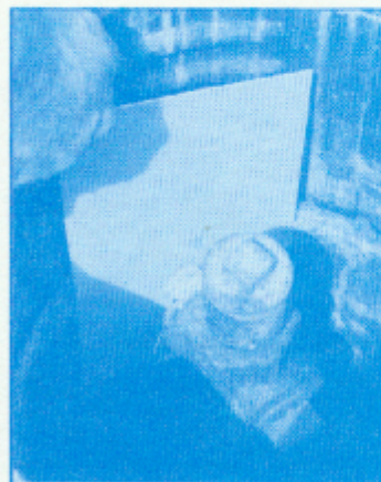
1/16" FRP FLATTIES being used to prevent contact between valve and metal curb box.
