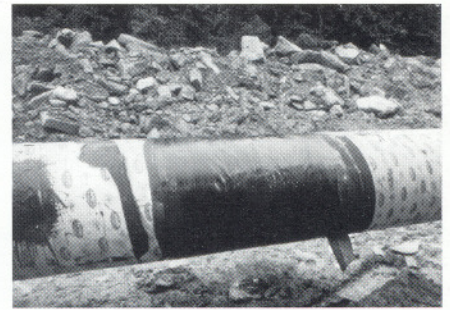
Finished application of Innercoat wax overwrapped with Guard-Wrap wrapper.
